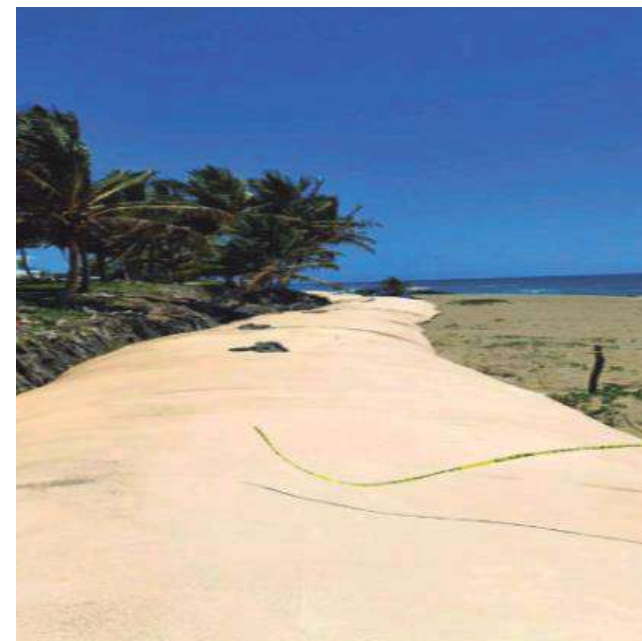
Geotube installation, Cabarete, Dominican Republic
