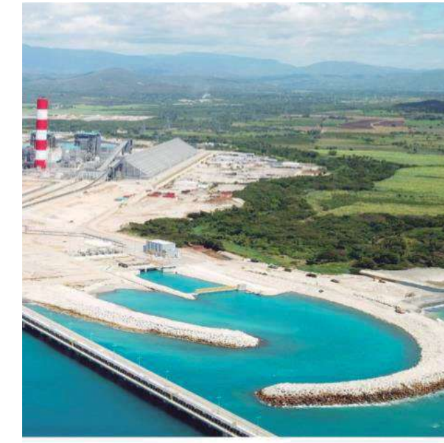
Breakwater for dock protection, Punta Catalina, Dominican Republic
