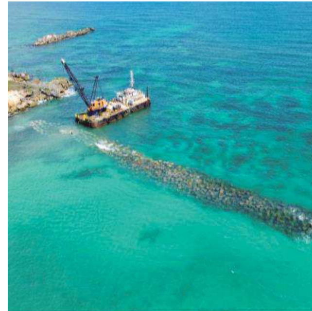
Breakwater protection at Cayo Levantado, Dominican Republic
